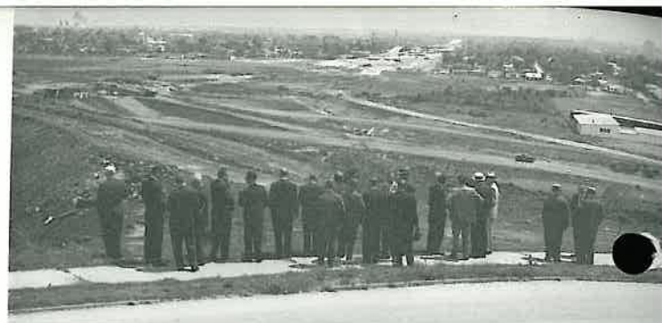
↑ The members of the tour are shown on Ark-Mo Drive in North Little Rock, surveying the North Terminal construction project.
